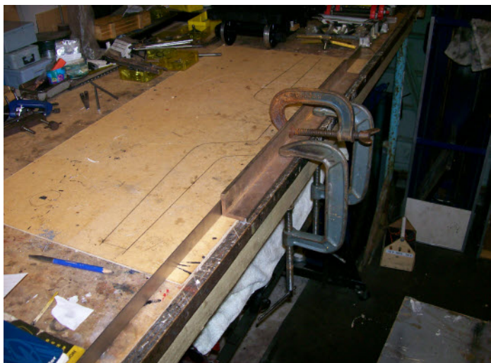
PhotoB - Set up to form Main Girder Flanges
