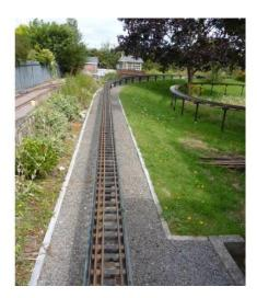
An assortment of second hand paving slabs had been acquired during the last year and has enabled the lining of the raised track cutting to be changed from timber boards to slabs
