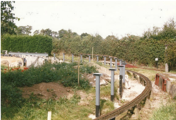
Track supports being installed at the tunnel end of the site
