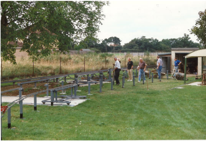
Steaming Bays under construction
